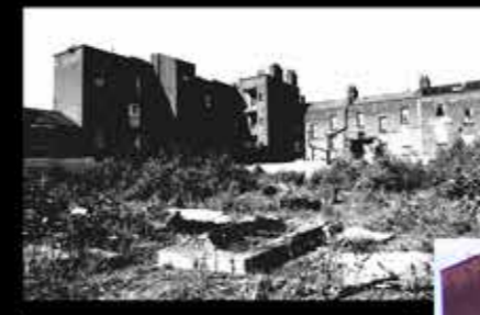
Derelict. In 1982 the garages that were on the site from early in the 20th century are demolished. The arch punched through no.10 Walnut Tree Walk for access is still there. These houses are empty and near-derelict. The floors and demolition debris from the garages are colonised by buddleia with a lot of fly tipping. Roots and Shoots will soon start to build what will become the Wildlife Garden.
